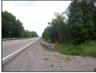
DRIVE LOOKING EAST
